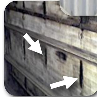
*Filter Rack directly in front of coils - arrows point to dirty coils caused by bypass between pleated filters.*
